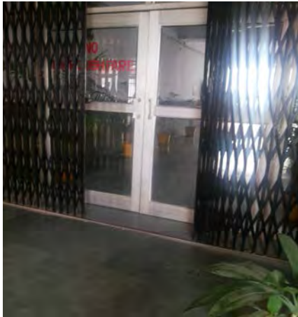
Fig 2.9 Picture: Doors complete covered by glass Panes
