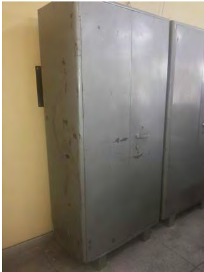
Fig 2.3: Cupboard near door capable of blocking exit
