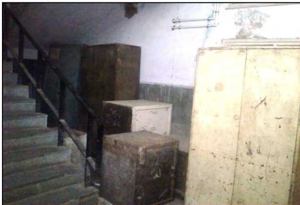
Picture: Material that cause blockage in exits
